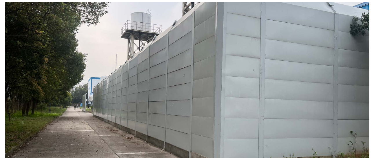
▲ Soundproof panels installed by NCC to reduce noise pollution
